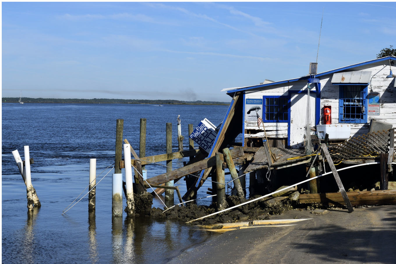
Damage from Hurricane Matthew
